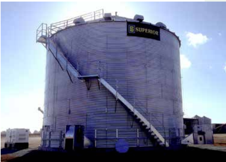
Drying Silo at Freemans Farms 2 x15kw Fans 13 vents Full Floor with "Bin Manager"
